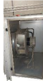
EC fans for AHUs, UFADs, Exhausts, DOAs
