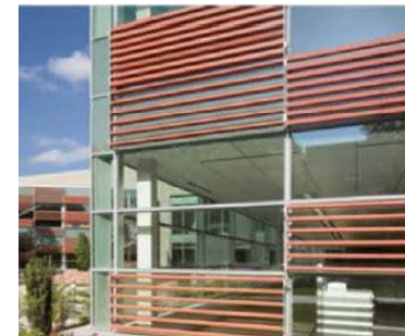
Double skinned Façade design to reduce heat ingress
