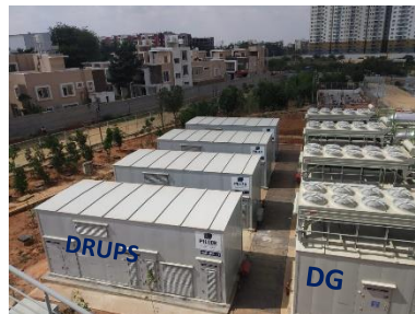
India's first Medium voltage Isolated parallel bus DRUPS system
